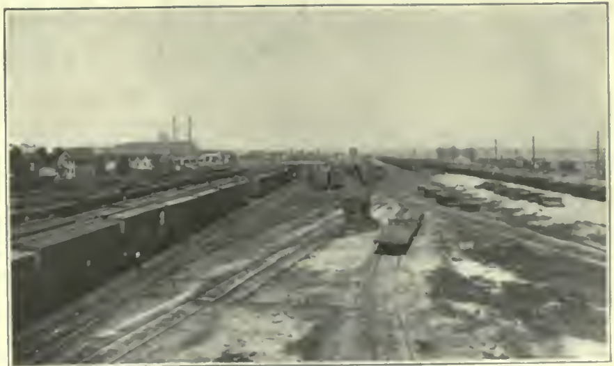
FIG. 336. FREIGHT YARDS. Hawthorne Yard of the Chicago, Burlington & Quincy Railroad.
